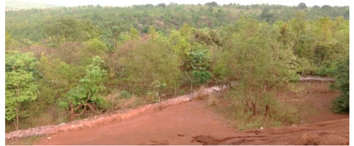
Retaining wall along with Plantations at the toe of dump slopes
