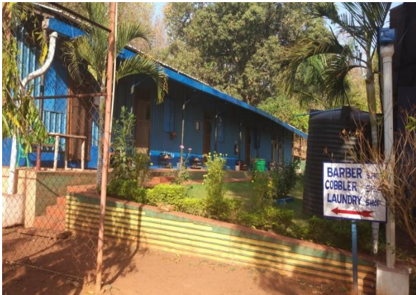
Roof top Rain Water Harvesting structure
